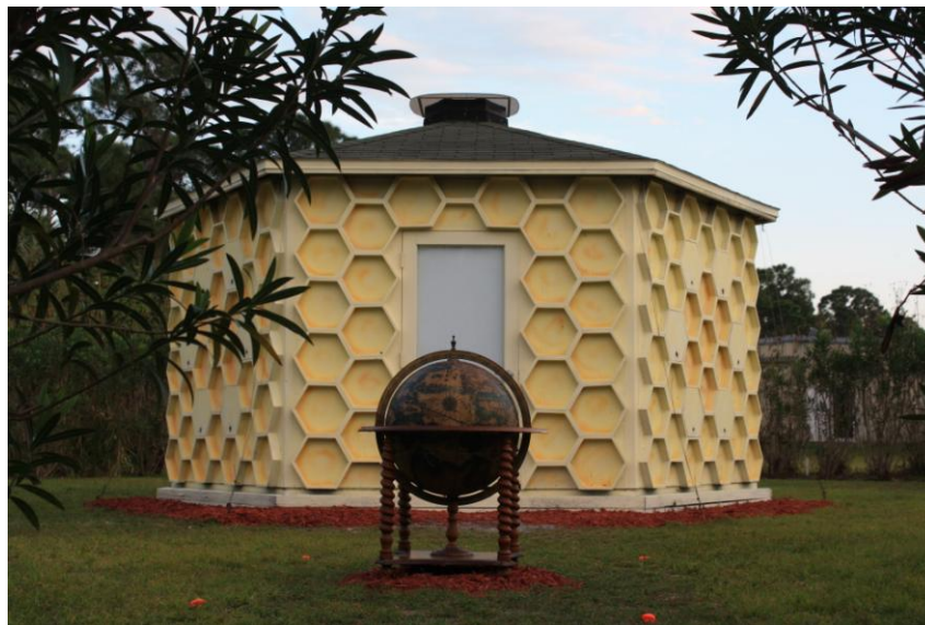
BeeRing's hut front side: Each of the six walls of the BeeRing© hut has six hexagonal-shape insertions that house six beehive habitats with open access for the bees from outside and a glass wall at the inside side to allow visitors inside the hut to appreciate the bee habitat .
